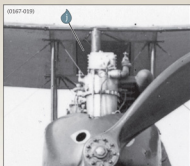
Gravity petrol tank detail from captured DH.9 B7620 A
